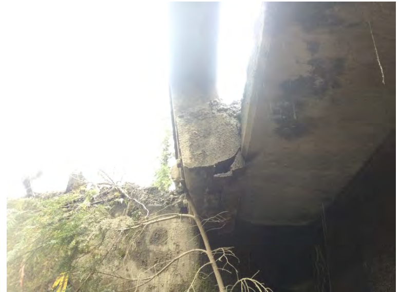
Downstream right bank side block
