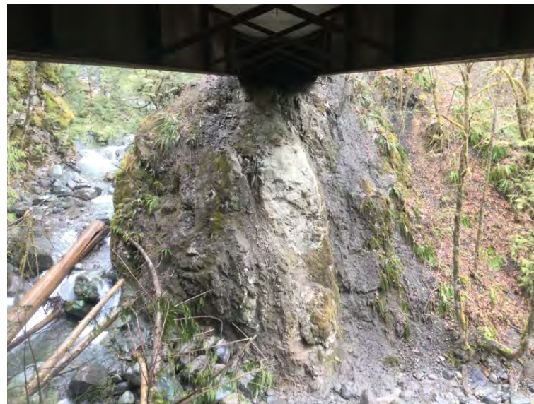
Left Bank Abutment when facing downstream
