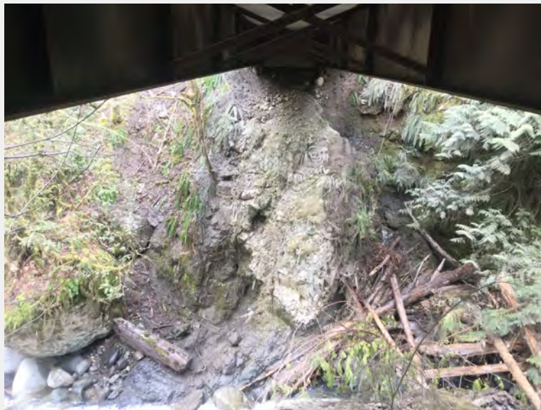
Right bank abutment
