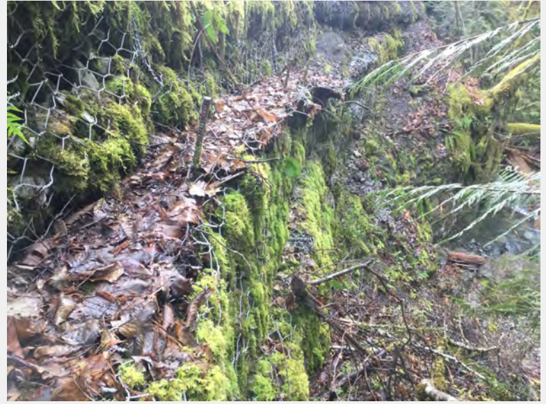
Upstream right bank gabions
