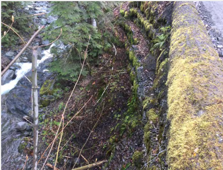
Upstream right bank gabions
