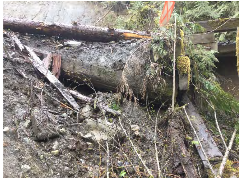
Downstream right bank fill retaining log condition
