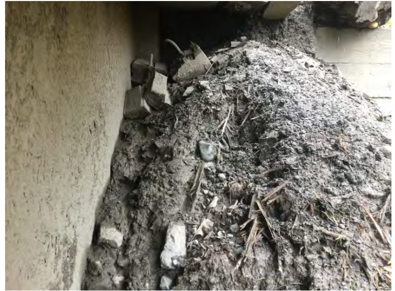
Fill against downstream left bank girder
